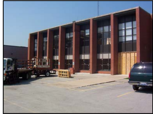
Typical enclosed walkway constructed to aid in the passage of students.
