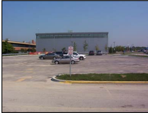
Parking lot constructed on the southeast corner of the facility.
